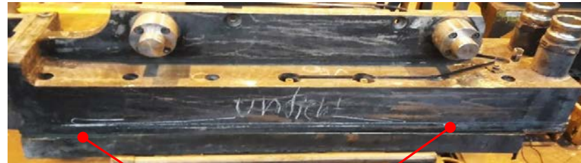
Leakage zone at the loose-side between copper plate and water box (length about 500 mm)
